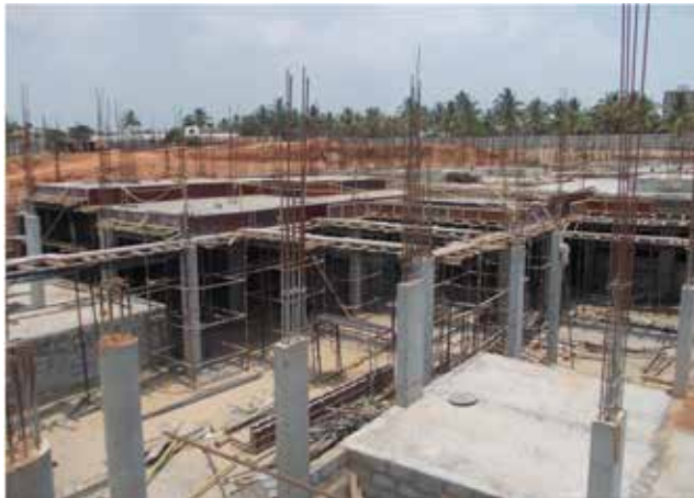
Super structure work of Villas in progress
