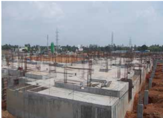
Completion of Basement for Villas
